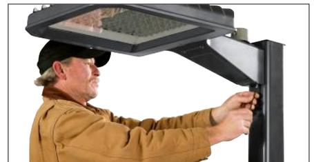
Tighten bottom bolts and complete wiring.
