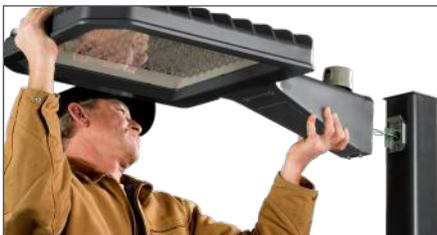
Remove existing fixture. Install cleat (or bracket) to pole.
