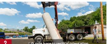
Lift pole base to vertical orientation.
